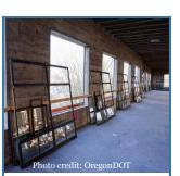
When replacing a whole window, it must comply with the IECC requirements for U-factor, SHGC and air leakage. When only replacing the glass in an existing sash and frame, the glass is not required to comply with the IECC.
