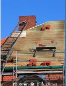
insulation does not completely fill the cavity, the exposed cavity is required to be "filled" with insulation. Note: insulation installed on a suspended ceiling with removeable tiles is not considered part of the minimum thermal resistance of the roof insulation. Roofs without insulation in the cavity and where the sheathing or insulation is exposed during re-roofing shall be insulated either above or below the sheathing.
