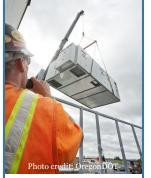
The replacement of an HVAC unit is required to comply with the IECC including minimum equipment efficiency requirements and equipment and system sizing.
